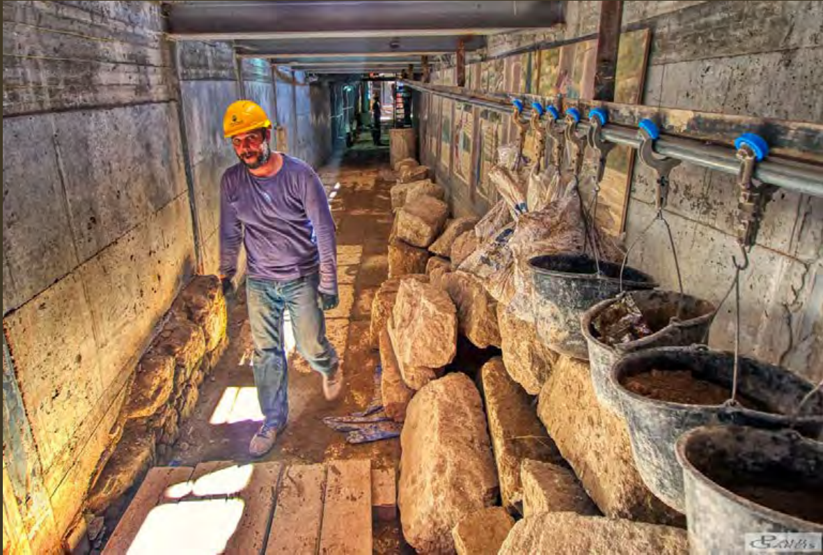
Tunnel Work Jerusalem
